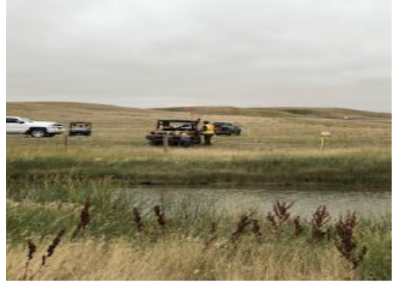
Heritage area being fenced in – km 161 + 000 – Aug 24, 2018
