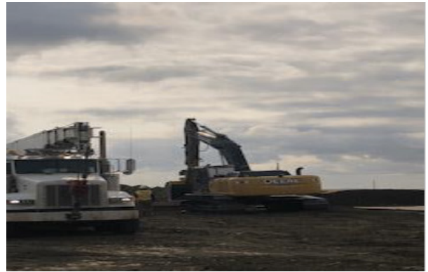
Excavator placing rig mats – km 252+100- Aug 25, 2018
