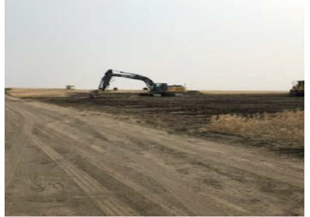
Excavator stripping topsoil – SF 160 – Aug 23, 2018
