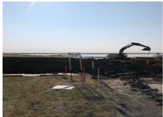
Digging slip bore pit – km 161+000 – Aug 21, 2018
