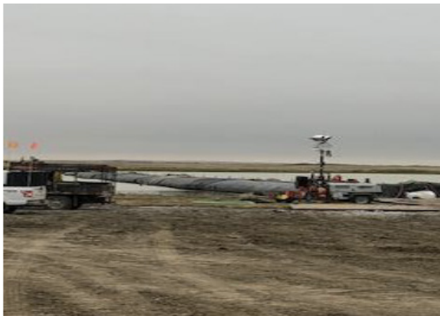
Aqua dam S.E– km 153+000 – Aug 24, 2018
