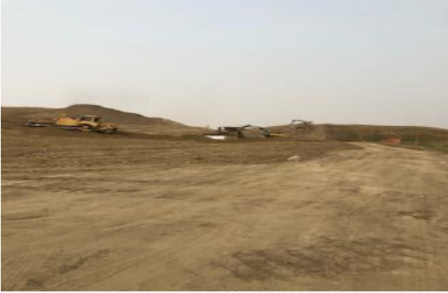
Hill being cut – km 220+900 – Aug 23, 2018
