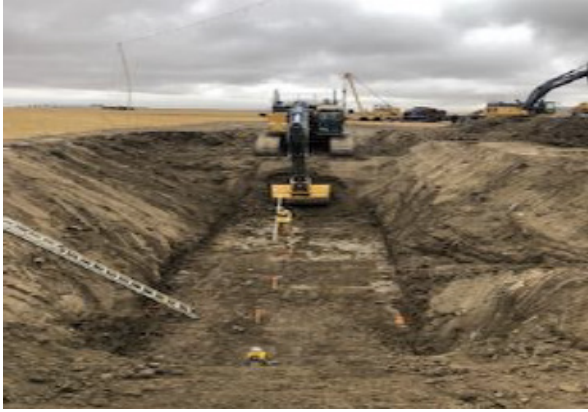
Bore bay digging – SF 115 – Aug 24, 2018
