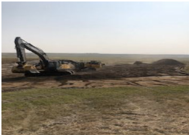
Excavator stripping topsoil – km 152+400 – Aug 20, 2018
