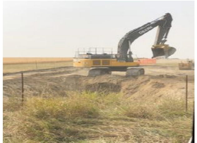
Excavator digging bell hole - km 172+039 – Aug 23, 2018
