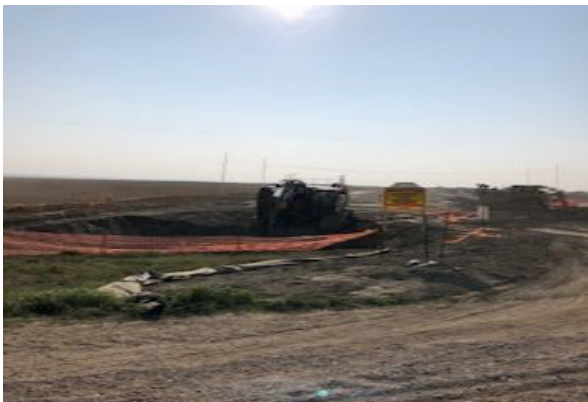
Excavator digging bell hole- Km 218+ 988– Aug 21, 2018
