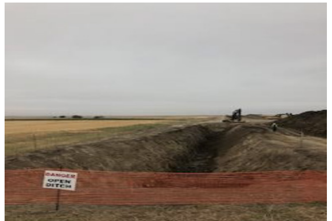
Excavator digging bellhole – km 150+000 – Aug 24, 2018
