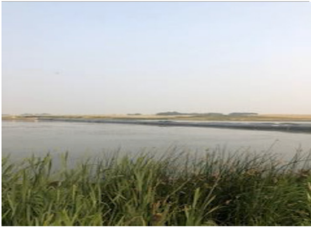
Aqua dam - km 165+265 – Aug 23, 2018
