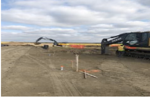
Excavators digging bore bays– Aug 25, 2018
