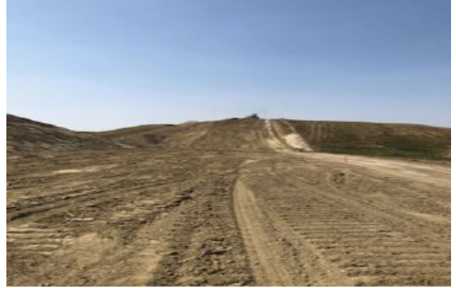
Access crew grading hill – km 222+800- Aug 25, 2018
