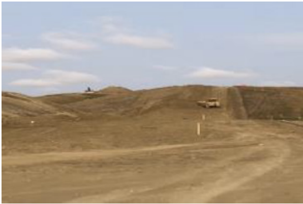
Dozer pushing dirt into valley – km 221+000 – Aug 25,2018
